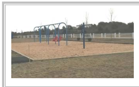
Phase 1 has been completed - Phase 2 has begun.
